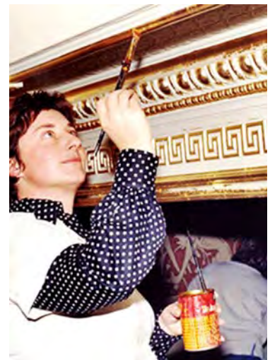
From top: the Legislative Assembly Chamber, circa 1980; a technician working on the restoration; detail from the restored Legislative Council Chamber; looking into the restored Legislative Assembly Chamber, as it appears today.
